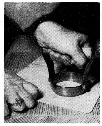
Hand Press Is Used To Cut Out Large Hosts
