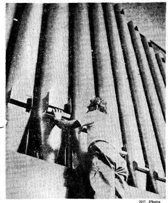
TREMENDOUS SIZE of the organ in the gallery above the main entrance to the National Shrine of the Immaculate Conception is easily seen when the size of the man in this photo is compared to that of the organ pipes. The pipe the technician is tuning is 32 feet high and weighs 825 pounds.
