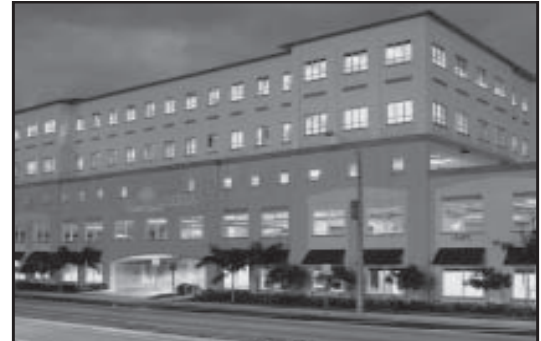
EAST HIALEAH CENTER 2475 East 5th Avenue
