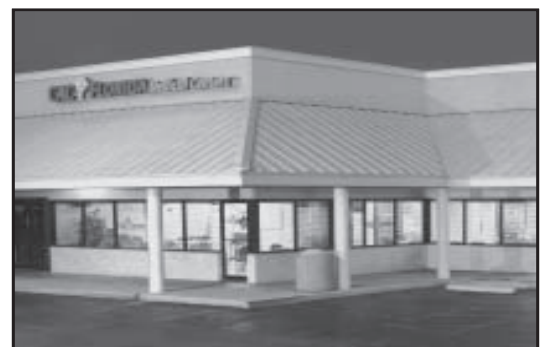
SOUTH DADE CENTER 18623 South Dixie Hwy
